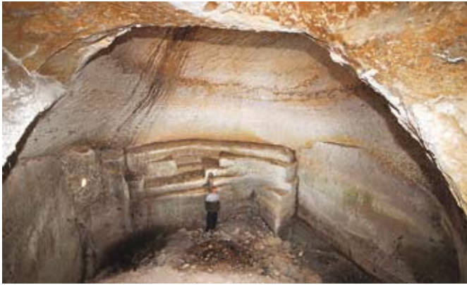
Fig. 7 - Signs of the end of quarrying, appear on the wall of a bell-shaped cave at H. Burgin: damaged blocks, scars and 'negatives', left on the walls after the removal of chalk blocks (photo B. Zissu).
